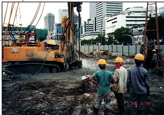
Stability improvement by use of tension piles and jet-grout base slabs.
